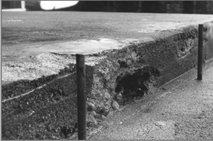
Repairs to Concrete Dock
