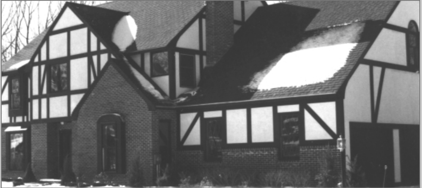
Stucco and Brick
