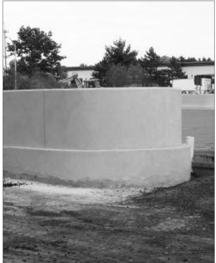
S&F Concrete, Inc., Natick Mall, Natick, MA
