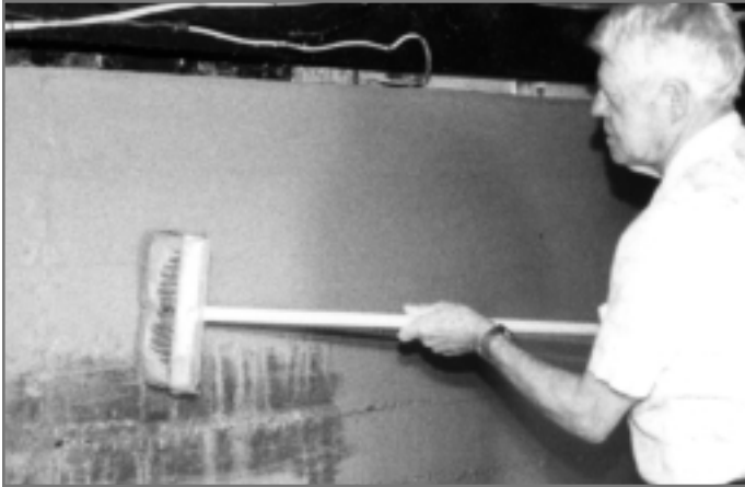
Interior Basement Application
