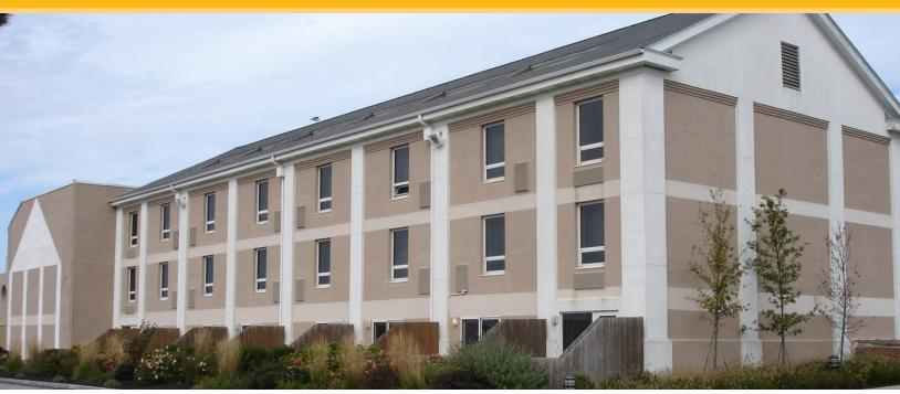
CALIFORNIA STUCCO<sup>TM</sup> is a Portland cement-based, water-resistant coating that is easy to apply and has the ability to withstand severe climatic conditions. It combines a great variety of textures with low maintenance cost in a permanent finish material. Available in white or gray. White CALIFORNIA STUCCO<sup>TM</sup> can be integrally colored with HAWK & TROWEL PIGMENT<sup>TM</sup>, available in 7 earth-tone shades.
